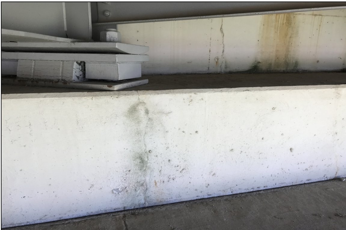
Abutment cracks
